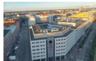
Yaskawa Europe GmbH, Environmental Energy Division, Helsinki, Finland
