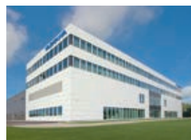
Allershausen, Germany Plant construction and robot systems
